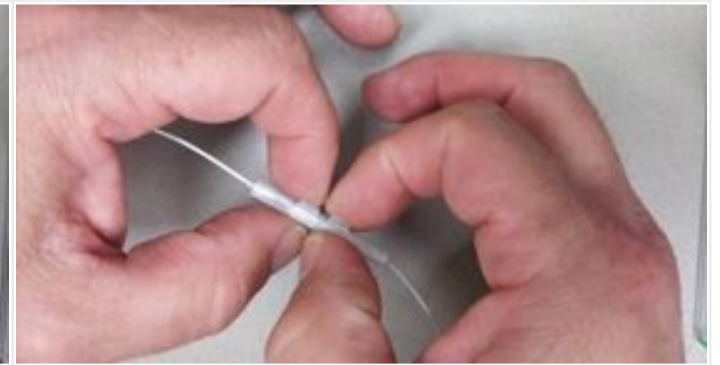
Then press down the middle connection tabs locking the fibers into place
