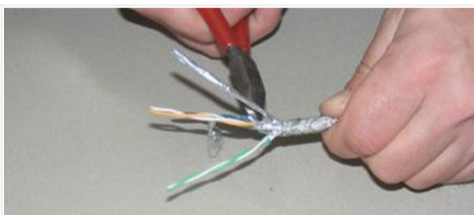
Separate the four pairs and remove the foil wrap from around each pair.
