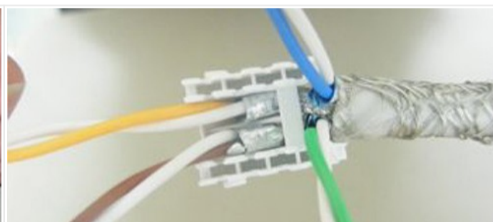
Insert front wires under the cross piece with the rear wires sitting at the back
