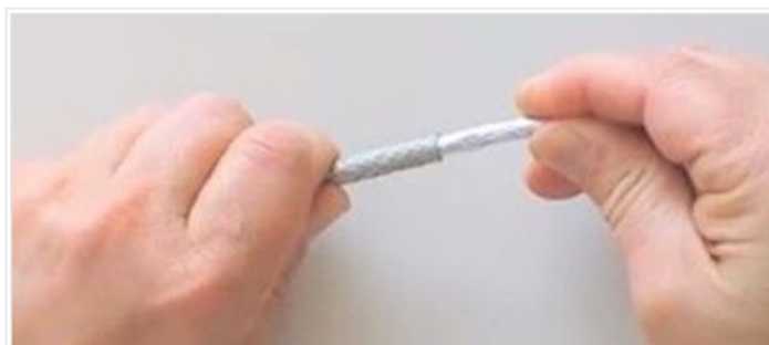
Strip 40mm of sheath from cable using stripper then roll back the braid onto cable so it is out of the way
