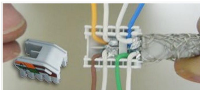
Press wires into the correct slots as per the color legend on the side of the cap
