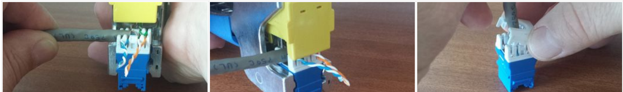
Squeeze handles together terminating and trimming wires
