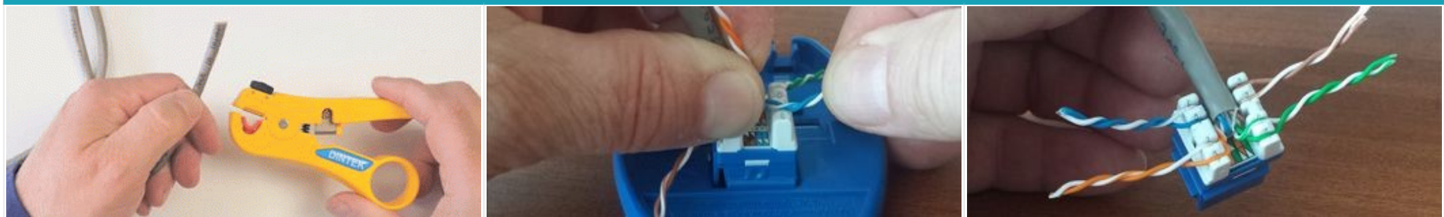
Strip 40mm of sheath from cable using stripper
