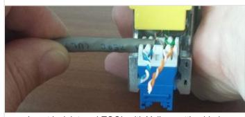
Insert jack into ezi-TOOL with Yellow cutting blade
