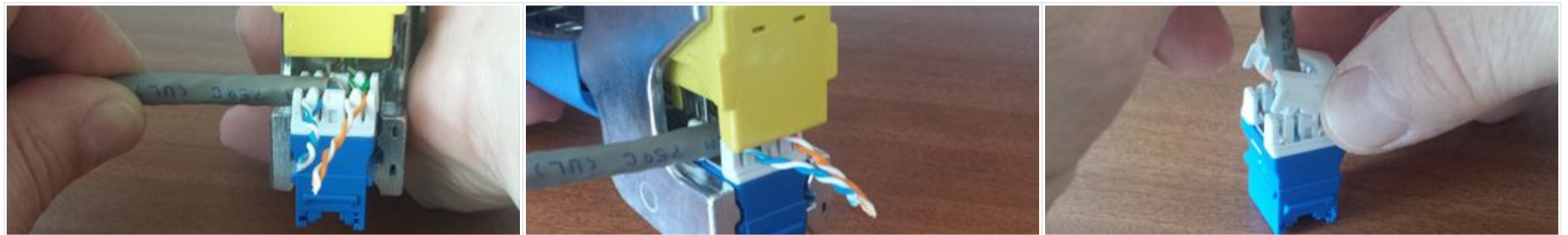
Insert jack into ezi-TOOL with yellow cutting blade
